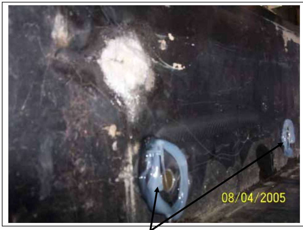
Silicone around drain tube holes then place drainpan in place. Ensure the drain pan holes are lined up with the box holes.
