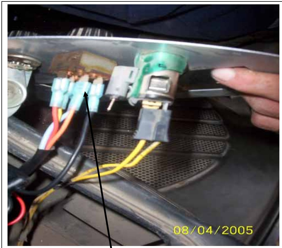
Wiring re connected to fan switch with female QD's installed.
